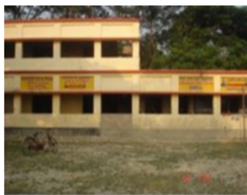
136/150 - Mayahouri F.P. School (Room No. 2)
