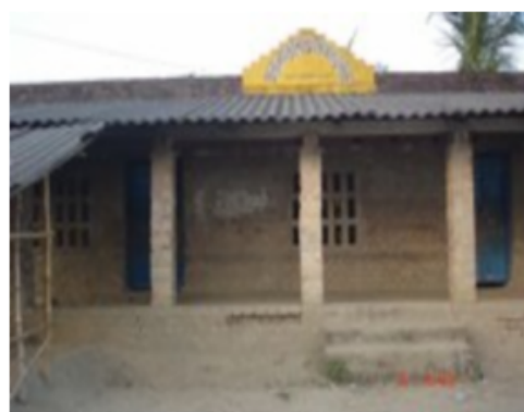
136/167 - Taranagar S.S.K. Building (Room -2)
