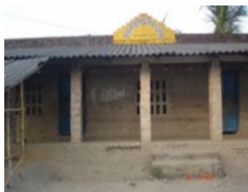
136/167 - Taranagar S.S.K. Building (Room -2)
