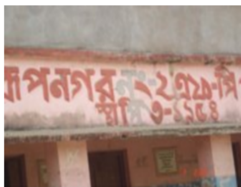
136/176 - Rupnagar No. 2 F.P. School (Room-2)
