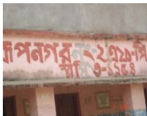
136/176 - Rupnagar No. 2 F.P. School (Room-2)
