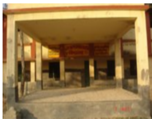
136/183 - Rupnagar F.P. School (Room-2)
