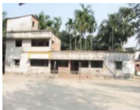
136/191 - Chuknagar F.P. School (Room No. 1)
