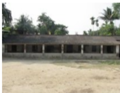
136/197 - Sahajadpur Chuknagar F.P. School (Room-2)
