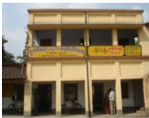
136/207 - Tulshighata F.P. School (Room No. 1)
