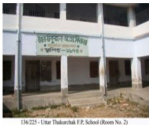
136/225 - Uttar Thakurchak F.P. School (Room No. 2)
