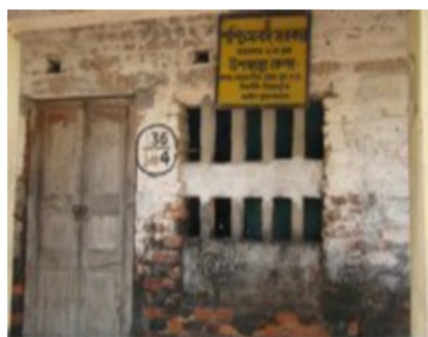
136/227 - Uttar Thakurachak Medical Sub-Centre (Room No. 1)
