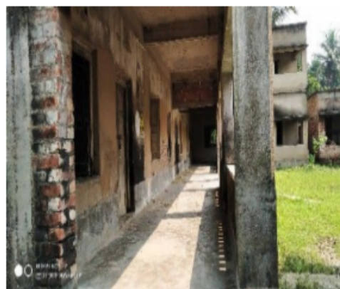
Polling Station Front View
