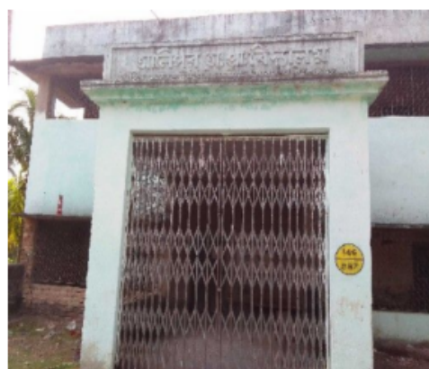
Polling Station Front View
