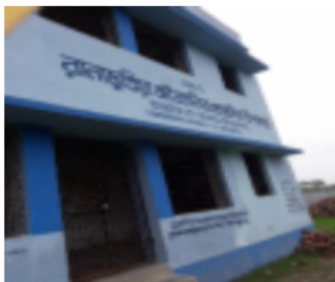
Polling Station Building Front View
