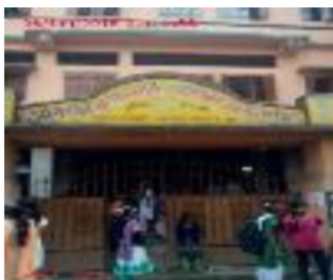
Polling Station Building Front View
