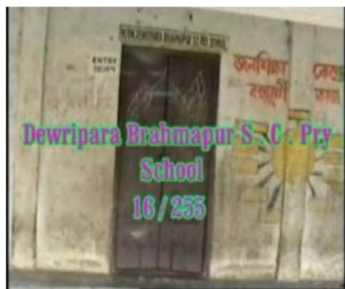
Polling Station Building Front View
