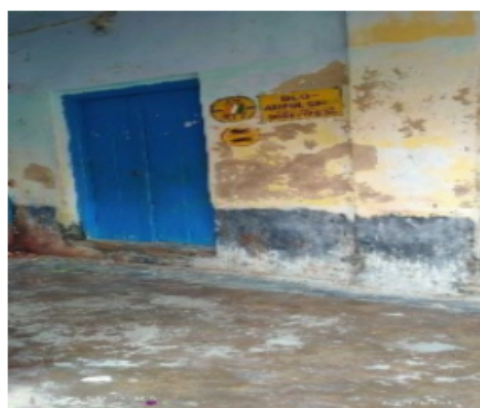
Polling Station Front View
