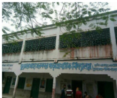
Polling Station Building Front View
