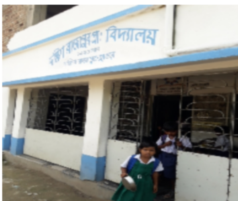
Polling Station Building Front View
