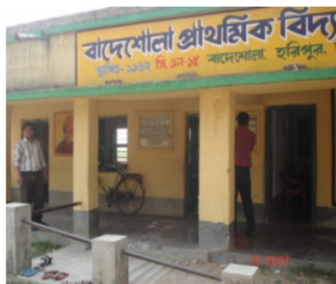
Polling Station Front View
