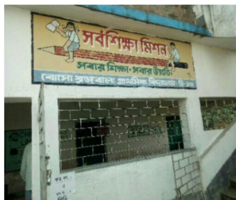
Polling Station Front View
