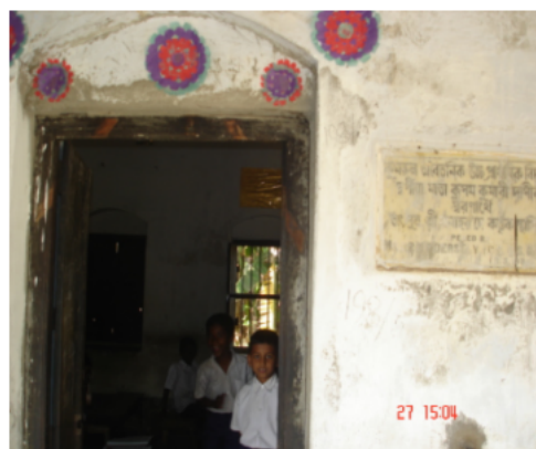
Polling Station Building Front View
