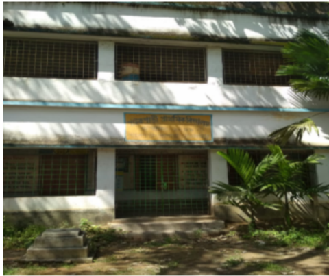
Polling Station Building Front View
