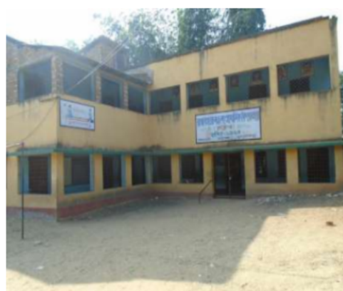
Polling Station Front View
