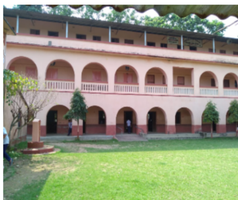
Polling Station Building Front View
