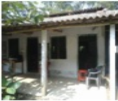
Polling Station Building Front View
