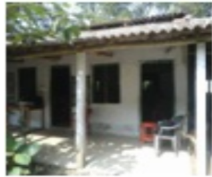
Polling Station Front View
