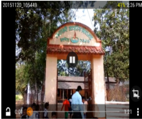
Polling Station Building Front View
