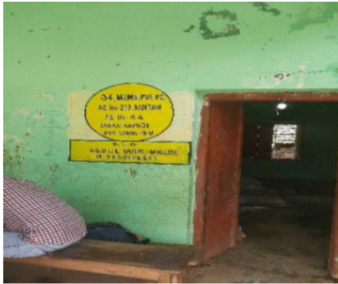
Polling Station Building Front View
