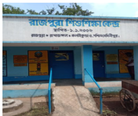
Polling Station Front View
