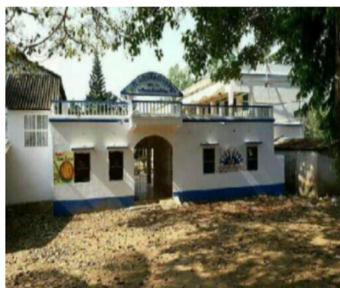
Polling Station Front View
