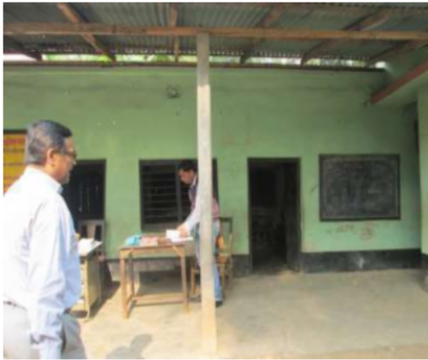
Polling Station Building Front View
