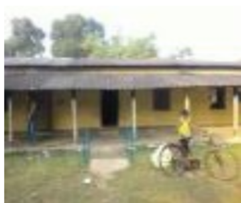
Polling Station Building Front View
