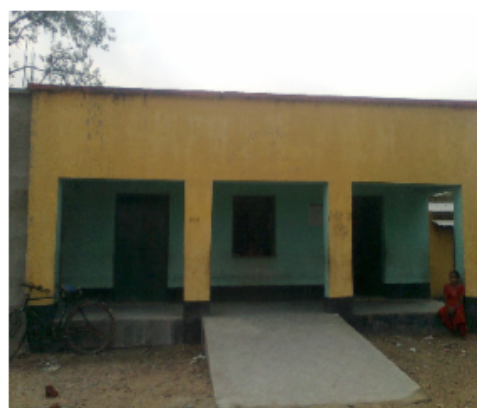
Polling Station Front View
