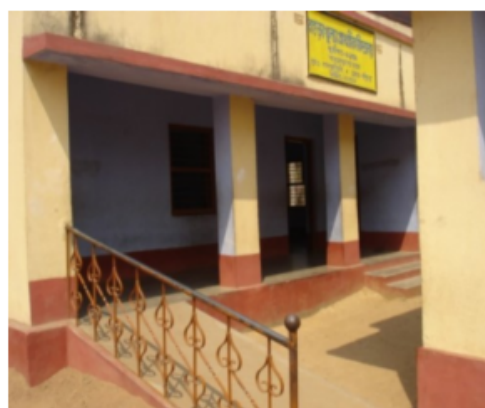
Polling Station Building Front View
