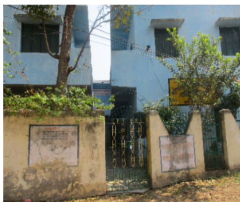
Polling Station Building Front View
