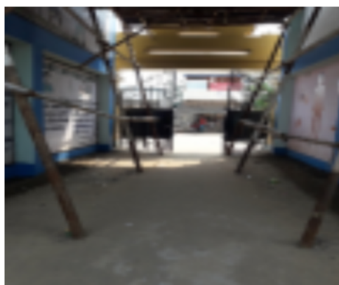
Polling Station Building Front View
