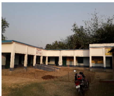
Polling Station Building Front View
