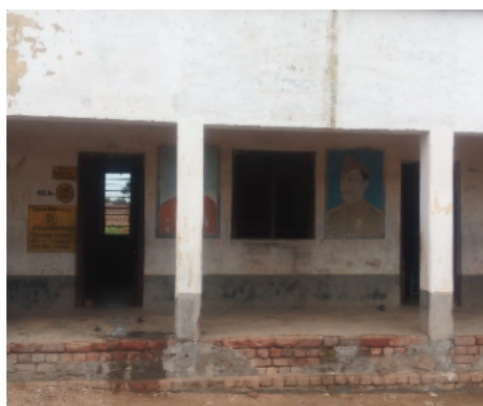
Polling Station Building Front View
