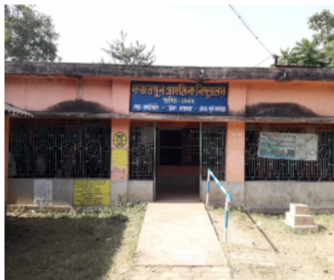
Polling Station Building Front View
