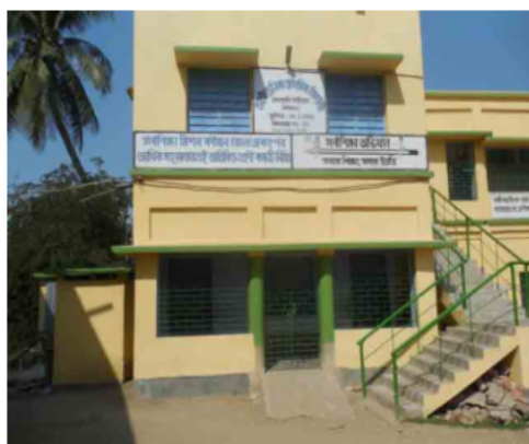
Polling Station Building Front View
