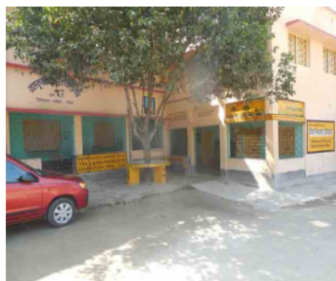
Polling Station Building Front View
