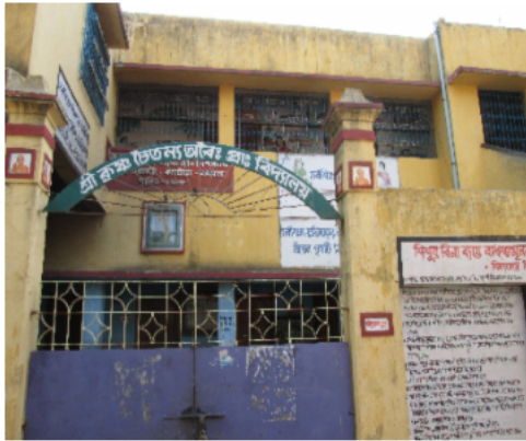
Polling Station Building Front View
