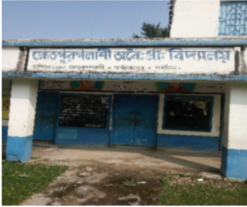
Polling Station Building Front View
