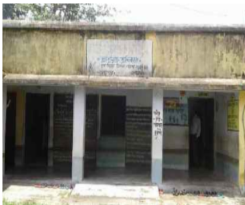
Polling Station Building Front View
