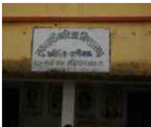
Polling Station Building Front View
