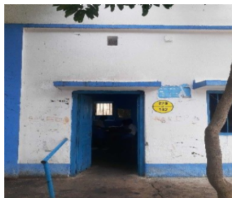
Polling Station Front View
