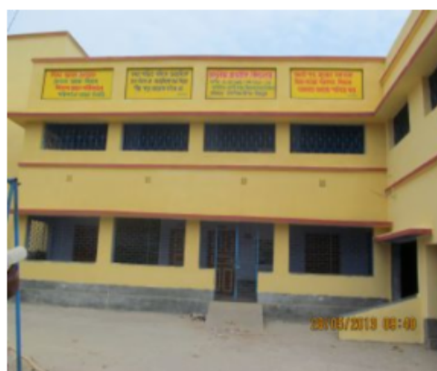
Polling Station Front View
