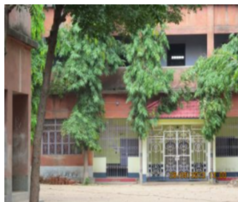
Polling Station Front View
