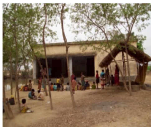
Polling Station Building Front View
