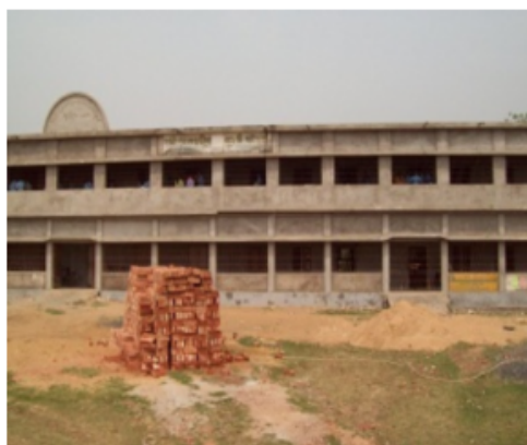
Polling Station Building Front View
