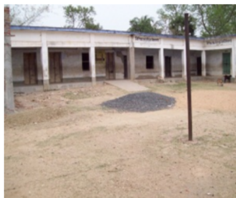
Polling Station Building Front View
