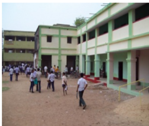
Polling Station Building Front View
